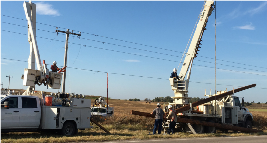
CKEC linemen work to replace a pole.
